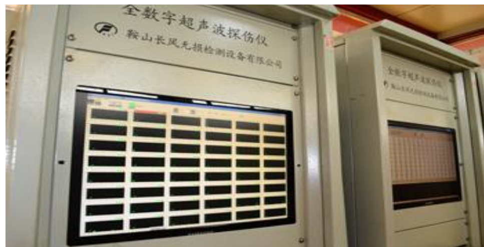
Continuous Monitoring Equipment of Ultrasonic Flaw Detection
